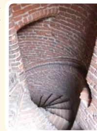
The brick staircase with ornate brick handrail
